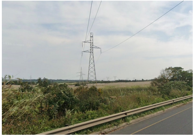
View south towards the site from the R34 with crossing of existing Impala-Zircon powerlines
